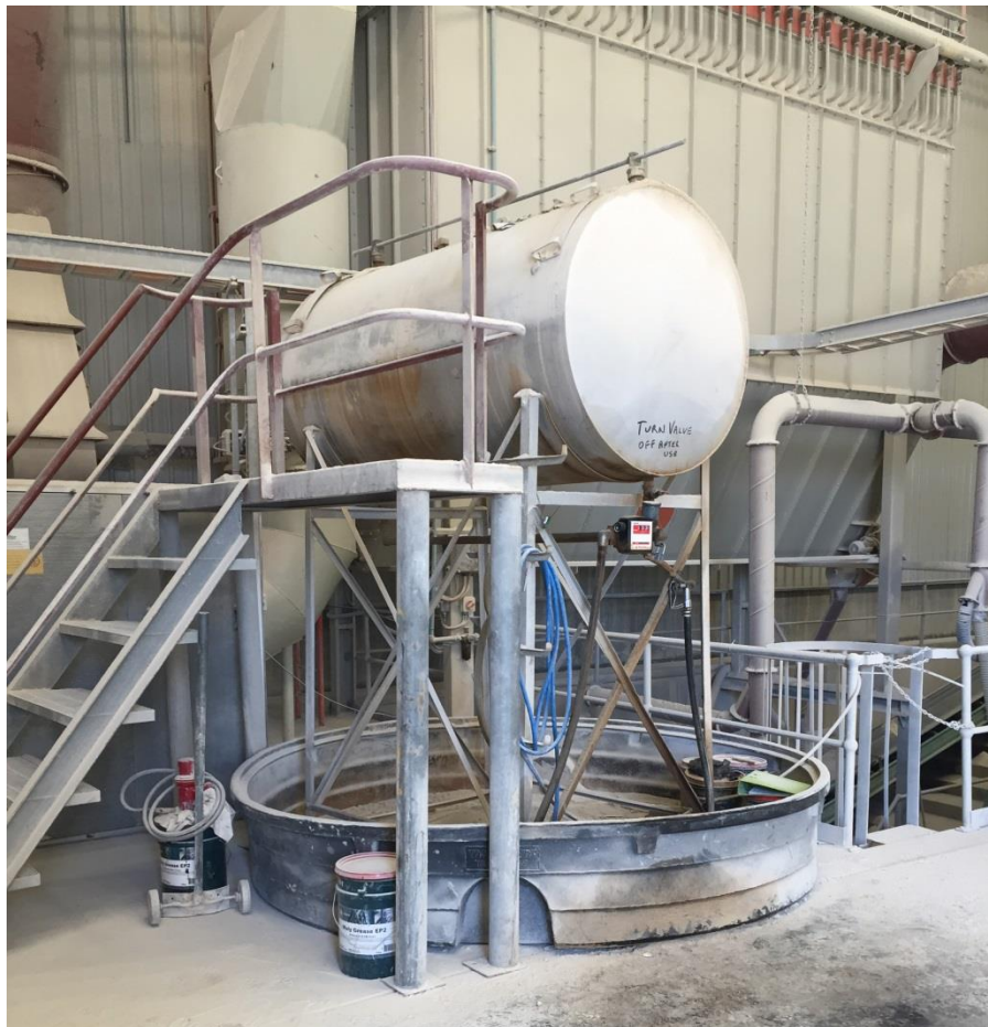
Photo 9. Bunded internal diesel storage tank.
