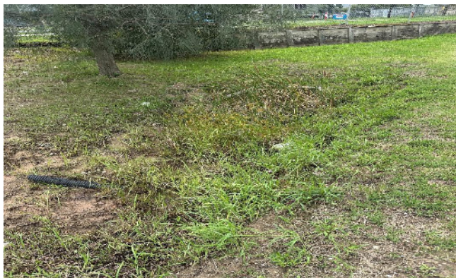
Plate 19 Culvert on northside of facility
