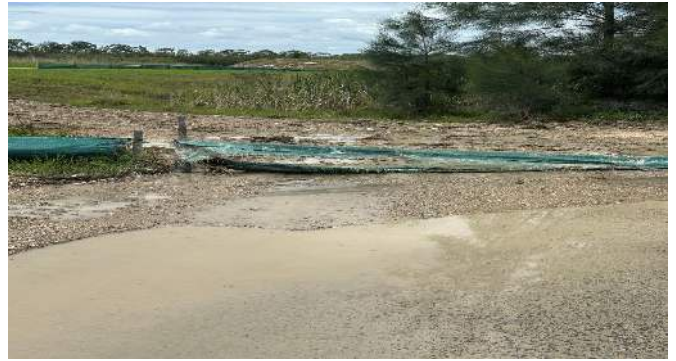
Plate 22 Sediment fence north of pond 1
