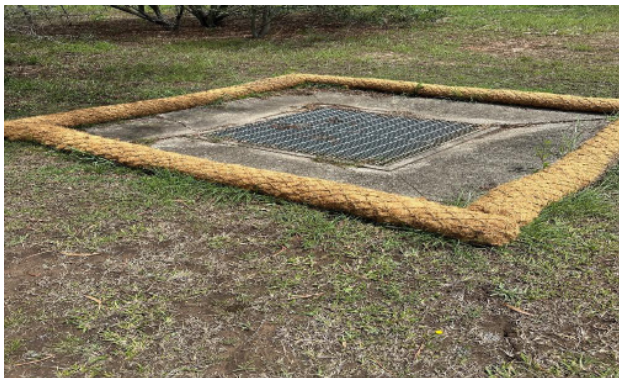
Plate 31 Stormwater drain with coir log
