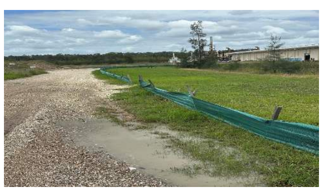
Plate 16 Sediment fence north of Pond 1
