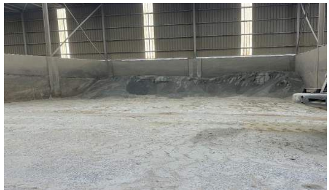
Plate 26 Raw Material storage (approximately 1200T capacity)
