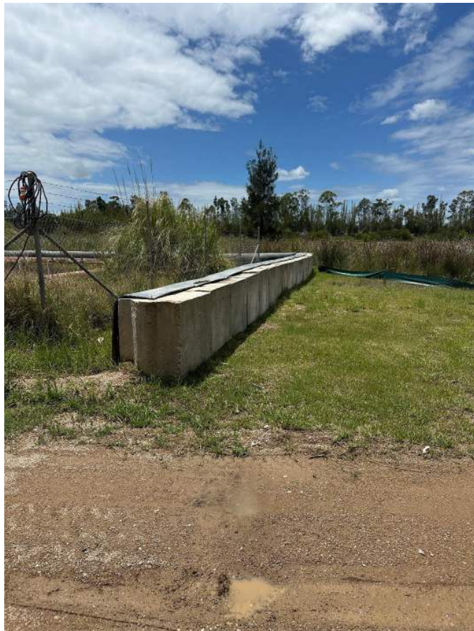
Plate 1 Aeration Pond additional barriers
