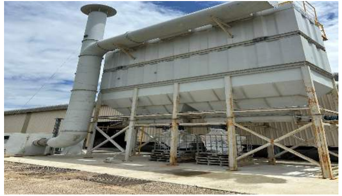
Plate 14 New Bag house Dust Bunded
