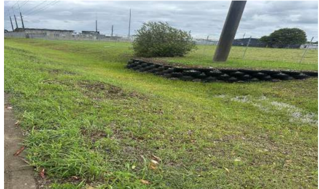
Plate 30 Water swale between driveway and substation following rain
