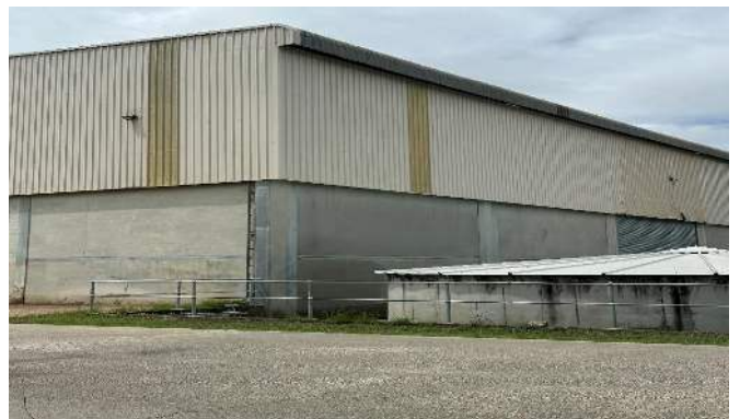
Plate 20 Factory lights reviewed in inspection
