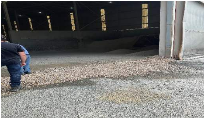
Plate 13 Broken Factory Roller Door (replacement ordered)
