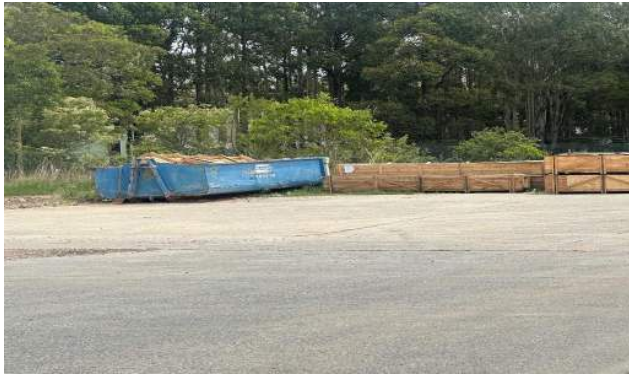
Plate 29 Timber waste sorting with a delivery of roller skins (additional timber skips stored after annual January delivery)
