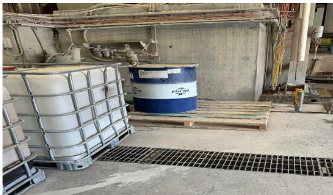
Plate 25 Lubricant stored by drain to aeration pond
